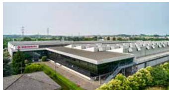
Giacomini S.p.A. Forging plant Castelnuovo del Garda (VR) (G3)
