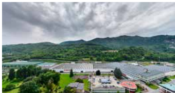
Giacomini S.p.A. Offices and brass machining San Maurizio d'Opaglio (NO) (G1)
